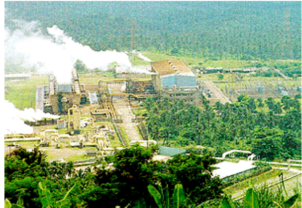
Makban plant complex in Laguna and Batangas
